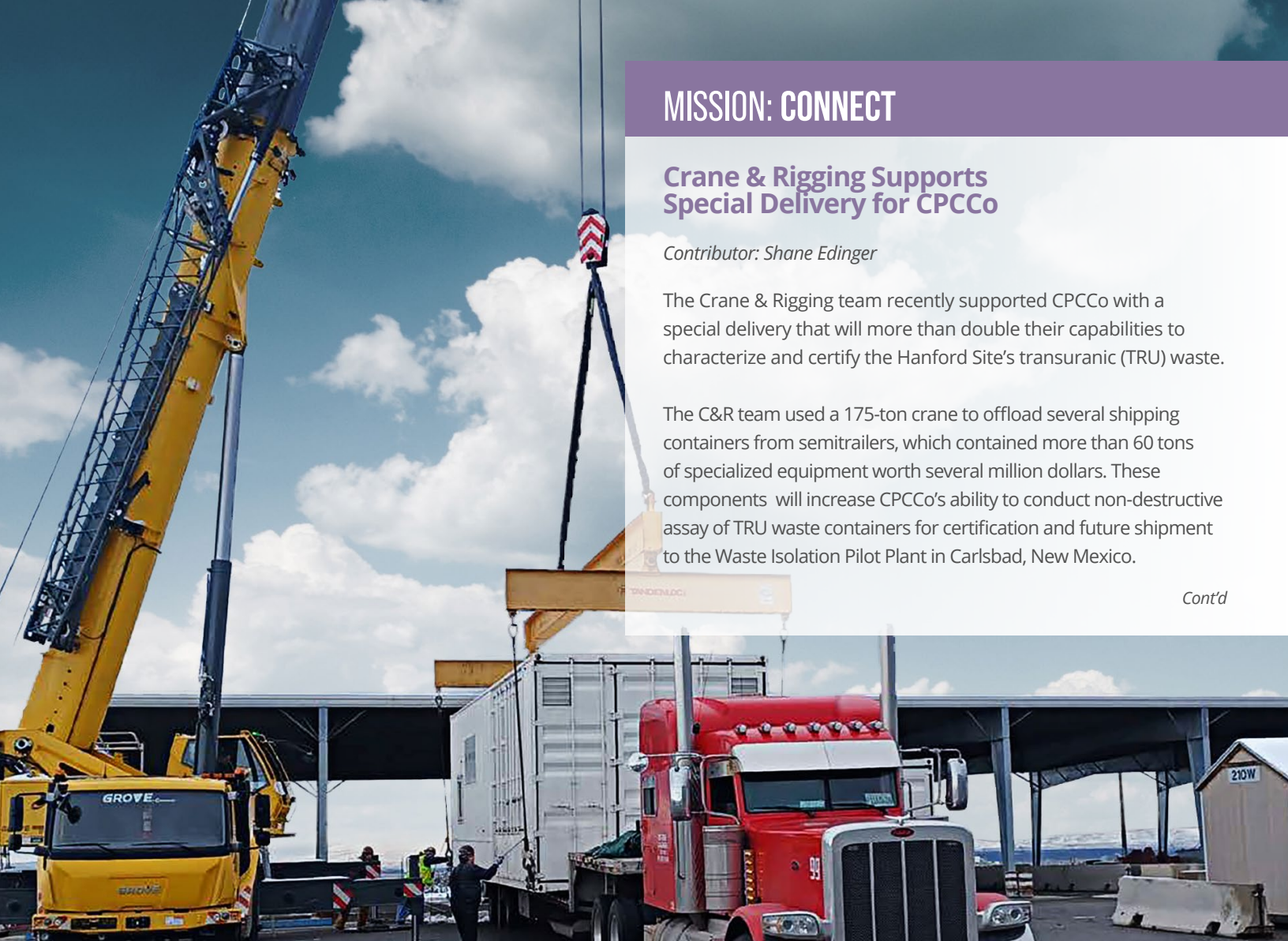
The Crane & Rigging team used a 175-ton crane to offload two large shipping containers loaded with specialized equipment to analyze transuranic waste. The container pictured weighed more than 62,000 lbs.
