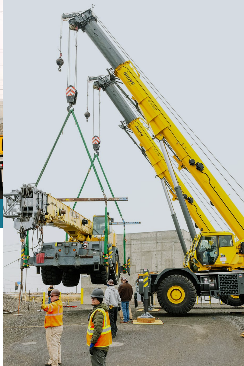
Crews prepare to guide the trailer beneath the lifted crane.
