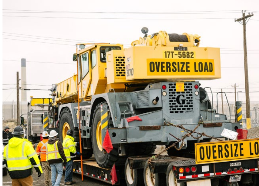
Crews measure the crane load's clearance before transport.
