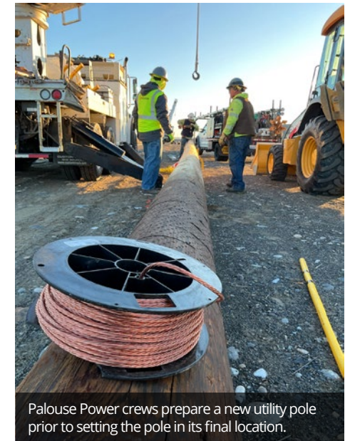
Workers with construction subcontractor Palouse Power replace a pole on 12 th Street as part of the Z-402 project.
