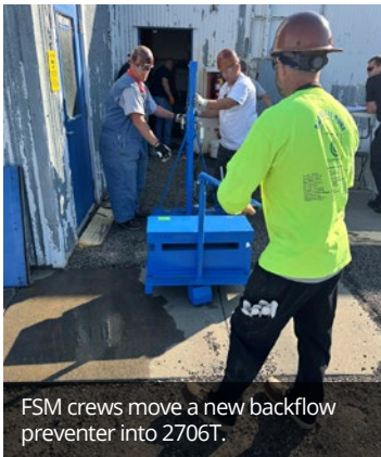
Matt Render and Derek Eves remove an outdated backflow preventer at 2706T.
