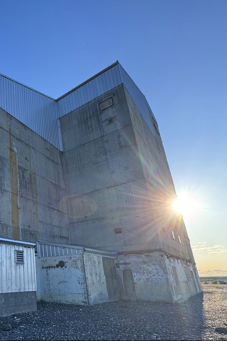
Hanford Site's C Reactor viewed from the south side prior to entry.
