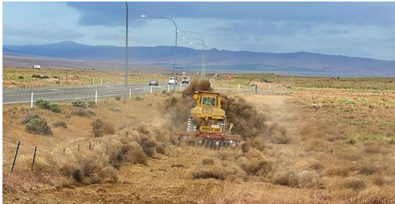
Heavy equipment operators clear accumulated tumbleweeds from the fire break line to make way for discing.
