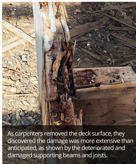
Carpenters remove decking at Inomedic Health Applications' onsite facility, exposing additional damage to the support structure.
